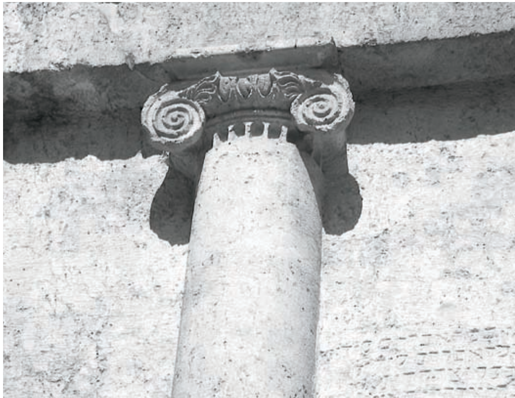
Fig. 7 The Ionic capital of the engaged columns on the western façade of the Tomb of Zechariah in the Kidron Valley, Jerusalem (Photo: O. Peleg-Barkat)
